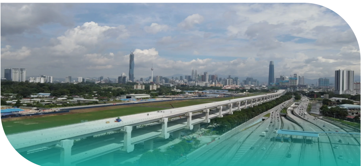
Gambar 34: Pembinaan deck slab di Seksyen 2 : Salak ke Pandan Photo 34: Construction of deck slab in Section 2 : Salak to Pandan
