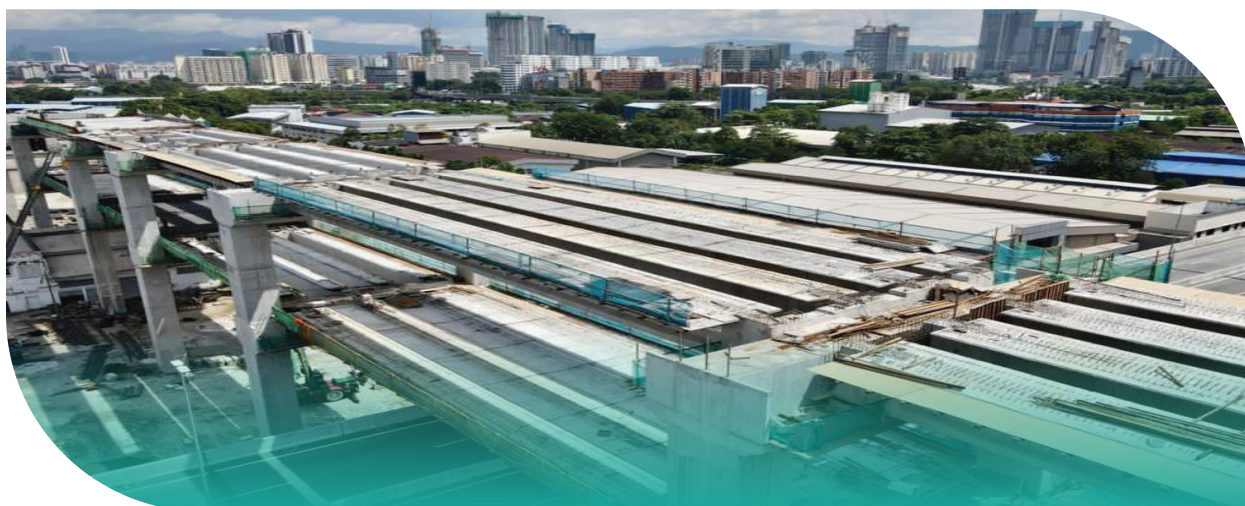
Gambar 39: Pemasangan rasuk di Seksyen 2: Salak ke Pandan Photo 39: Beam installation works at Section 2 Jalan Chan Sow Lin in Section 2 : Salak to Pandan
