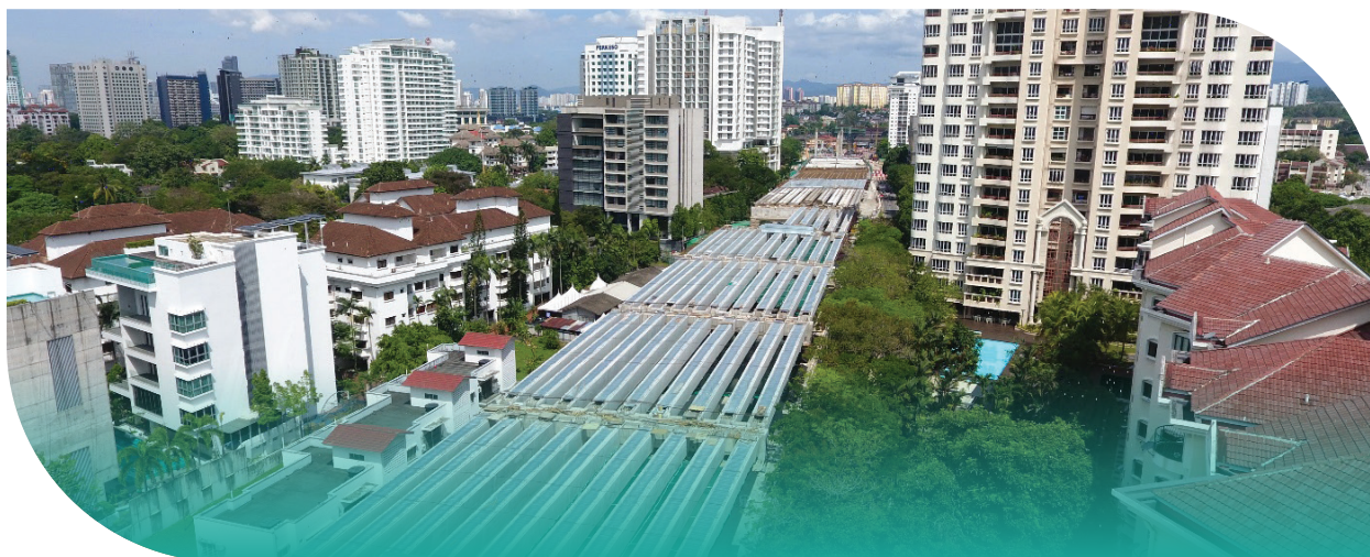
Gambar 37: Pemasangan rasuk di Seksyen 2: Salak ke Pandan Photo 37: Installation of beams in Section 2: Salak to Pandan
