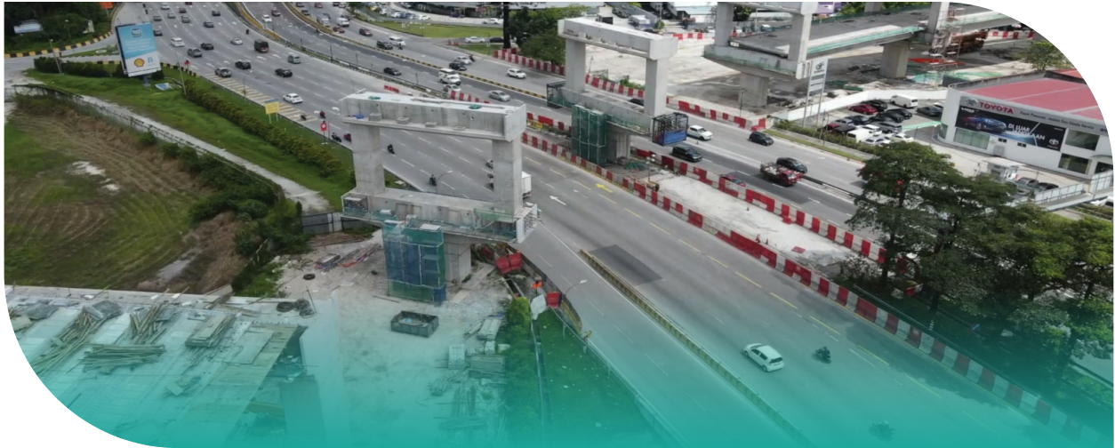
Gambar 35: Pembinaan Struktur Pier Cross Head Di Seksyen 2 : Salak Ke Pandan Photo 35: Construction of Pier Cross Head structure in Section 2: Salak to Pandan
