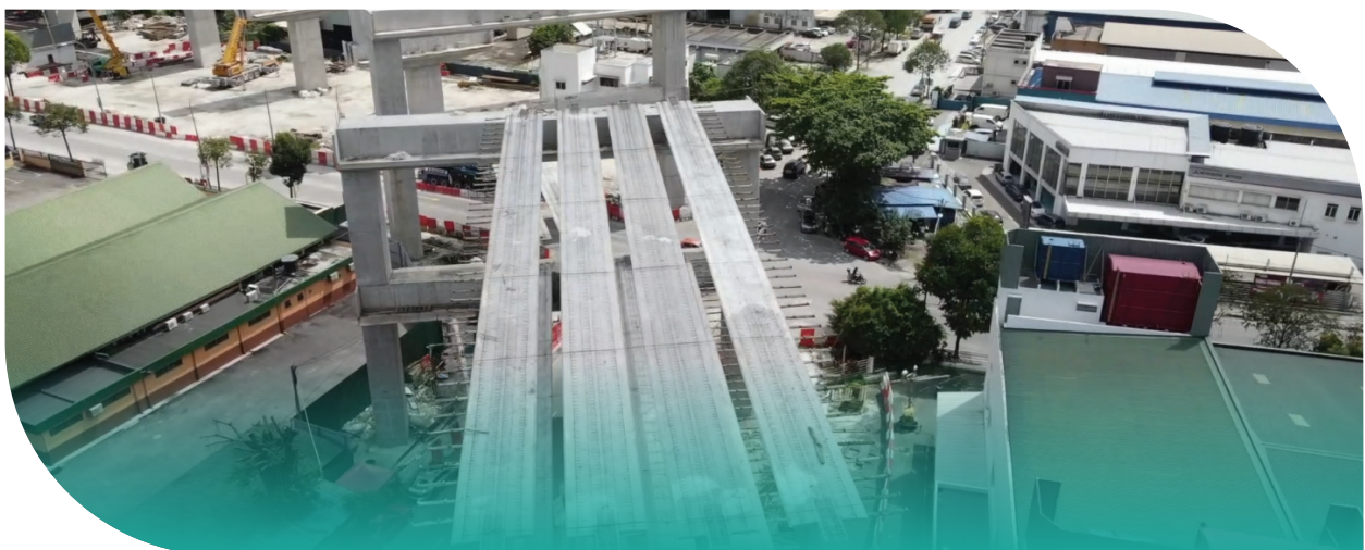
Gambar 36: Mengangkat Struktur Rasuk di Seksyen 2 : Salak ke Pandan Photo 36: Carrying Beam Structures in Section 2: Salak to Pandan
